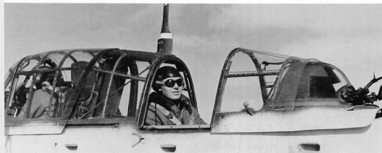
A close up view of the canopy of a Ju 87 D, almost certainly of II./St.G 3, showing the pilot and gunner in their positions, although the latter lacks armament; only the sights for his MG 81Z are in place. The stencilling on the aerial mast reads 'Vorsicht-Nicht Anfassen': 'Caution – do not touch'.
