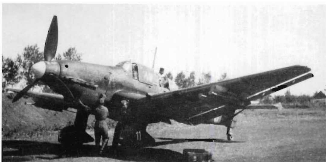
A Ju 87 D-3 of I./St.G 2. Note the aircraft letter L and the numeral 11 on the undercarriage fairing. When Gruppen consisted of three Staffeln, some letters were not used in aircraft code systems, hence the slight mismatch between the L, the twelfth letter of the alphabet, and the 11.
